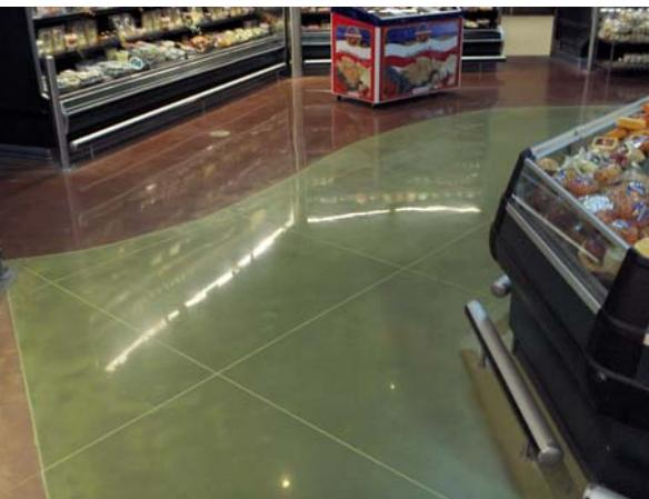
Staining and sealing concrete produces a natural look and feel with less maintenance than many other floor coverings, although unpolished surfaces will require an occasional re-sealing.
